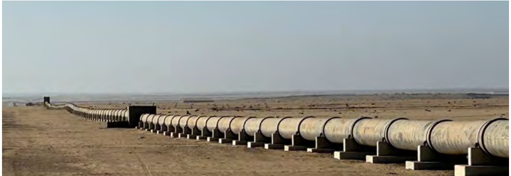
Figure 135: Connecting the water source with the distribution centre [Source: D von Oertzen]
