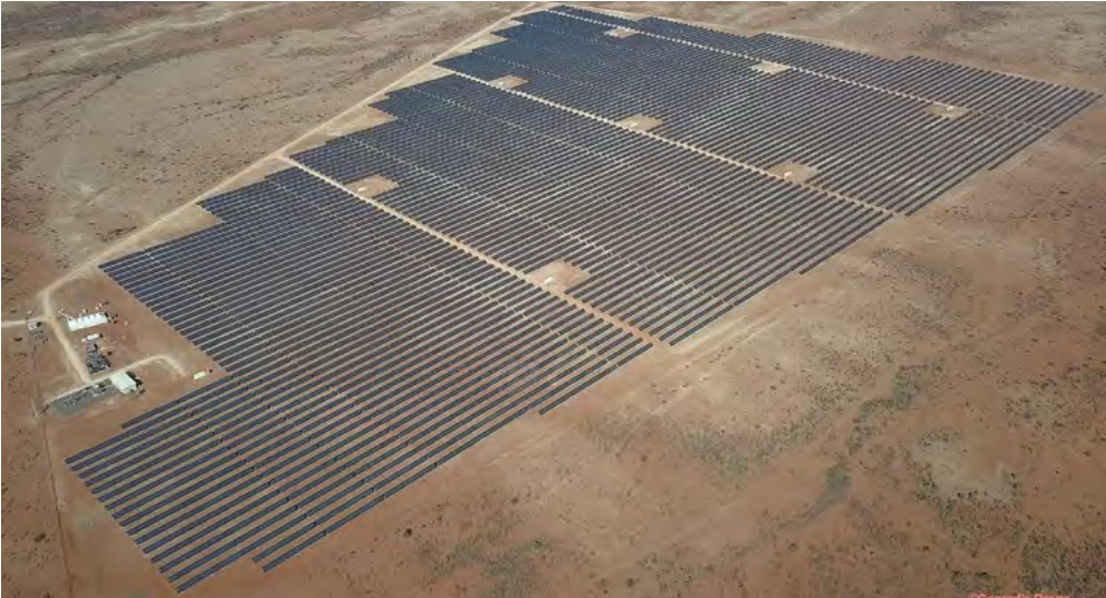
Figure 74: The 37 MW Alten solar PV plant east of Mariental [Source: C Roedern]
