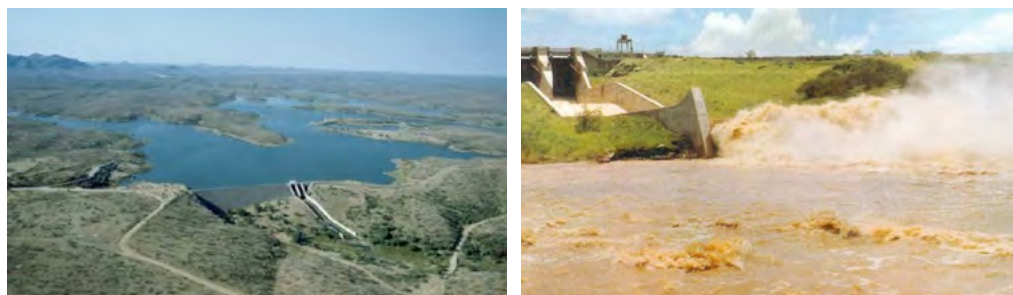
Figure 37: Von Bach Dam (left), and the Von Bach Dam spilling (right) [Source: DWA]
