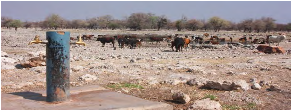
Figure 15: Water supply infrastructure in central-northern Namibia [Source: G Schneider]
