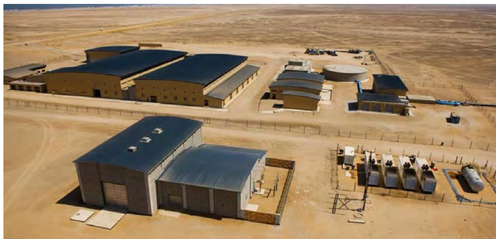
Figure 133: The Erongo Desalination Plant [Source: Orano]
