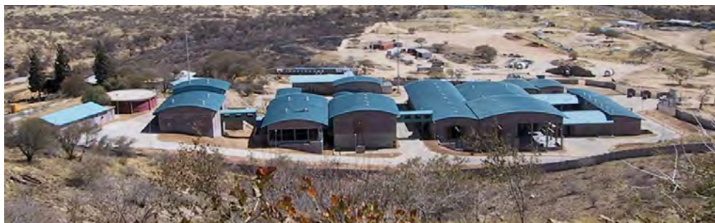
Figure 11: Windhoek's water reclamation plant [Source: P Heyns]
