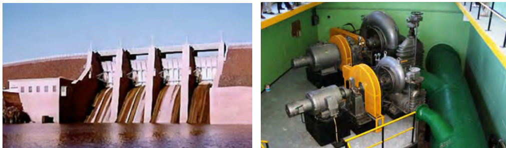
Figure 47: Hardap Dam (left) with hydropower turbines and generators [Source: P Heyns]
